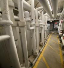
Figure 2. Piranha System Installed at the Seven35 Building (left) and the Hot Water Piping at the Seven35 Building (right)
