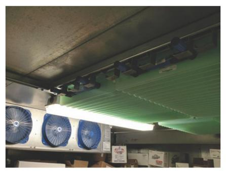
Figure 6. Salt-water PCM Application (Source: Viking Cold Solutions)
