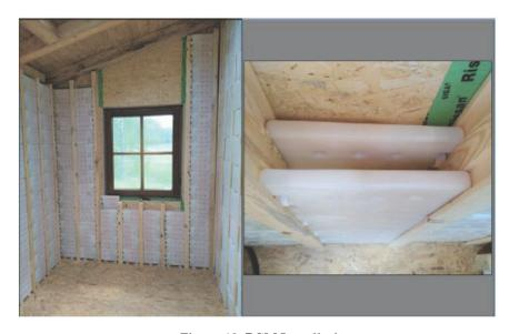
Figure 12. PCM Installation
