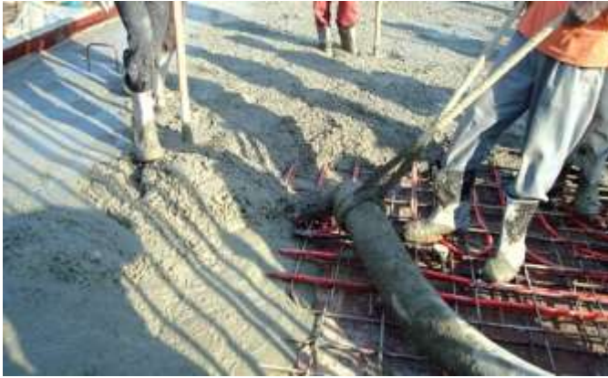
FIGURE 5: CONCRETING OF SLAB WITH RADIANT PIPES
