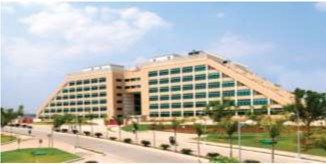
FIGURE 1: SDB-1 BUILDING, HYDERABAD
